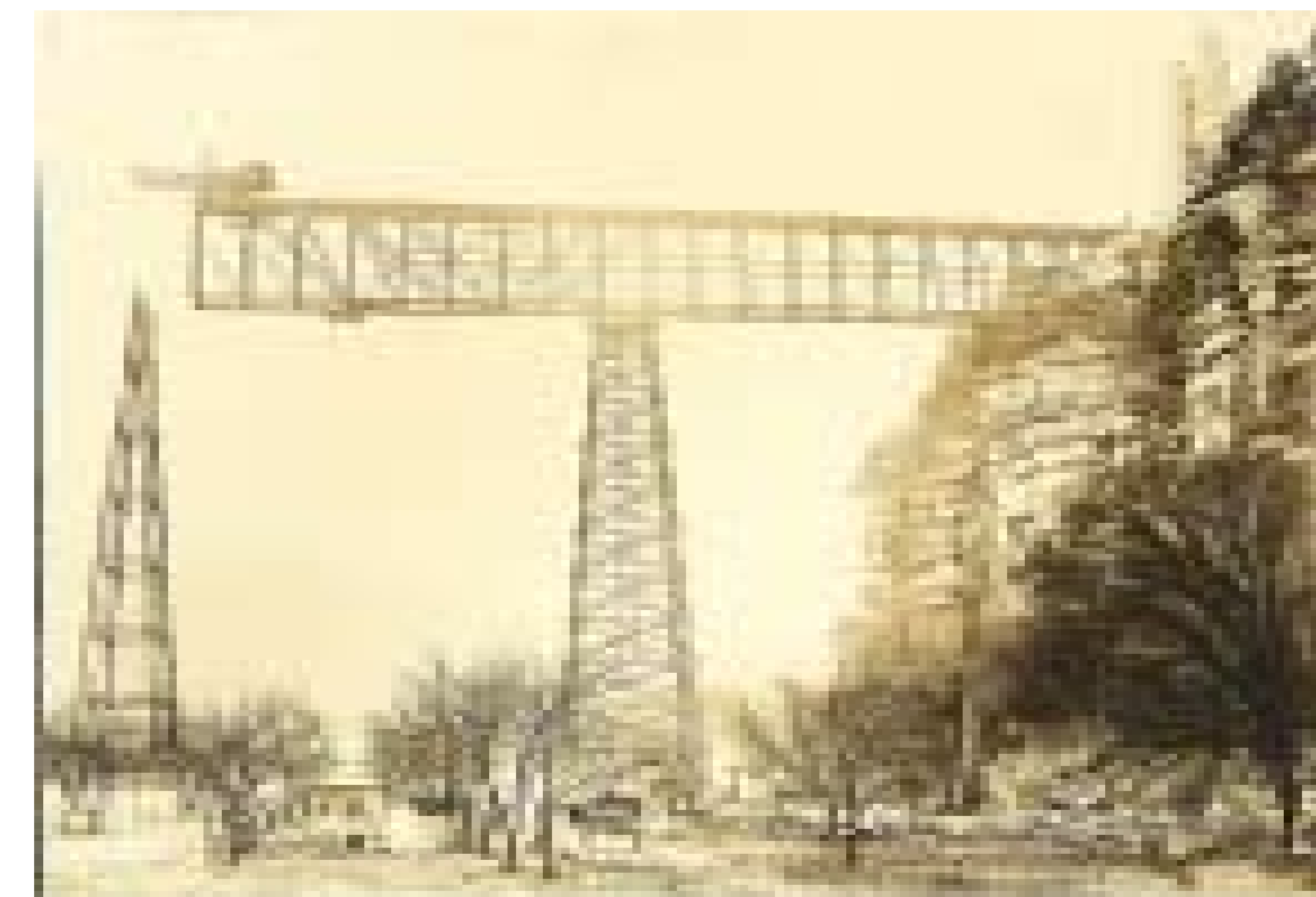
Construction at High Bridge in 1877. Note the temporary wooden towers.
