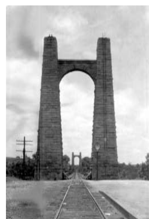
Shaler's cantilever bridge did not require the stone towers, but still they remained.
