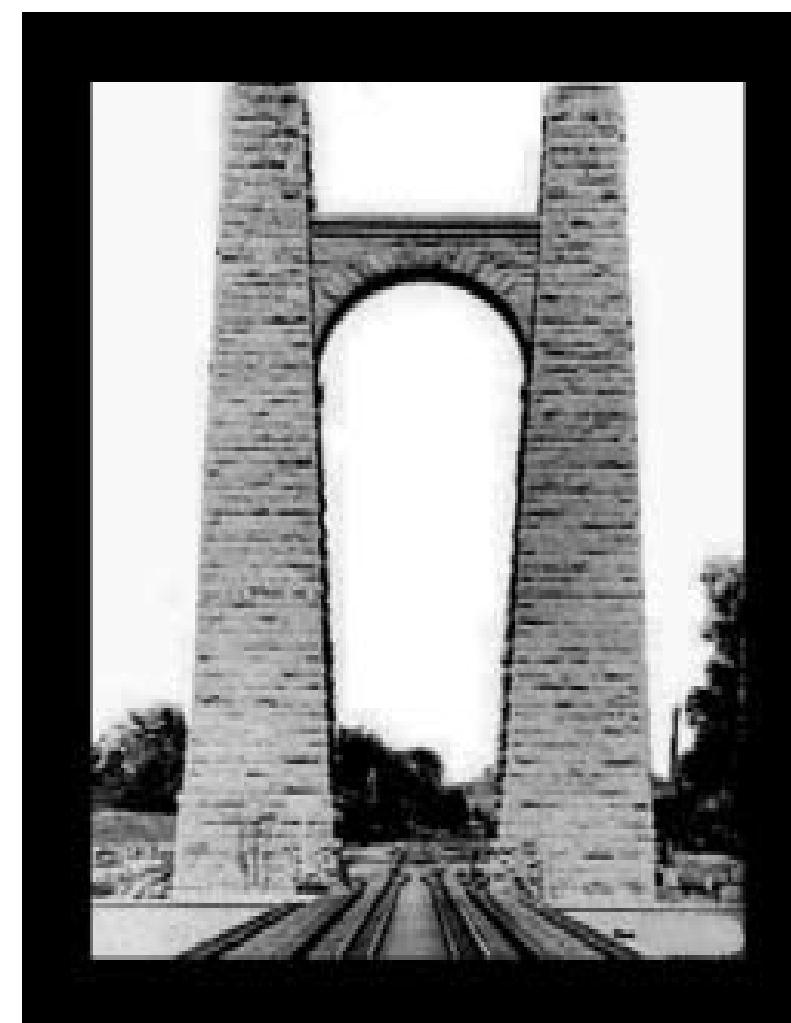
Roebling's stone towers, which were built to support the steel cables of a suspension bridge, graced the cliffs of the Kentucky River for
